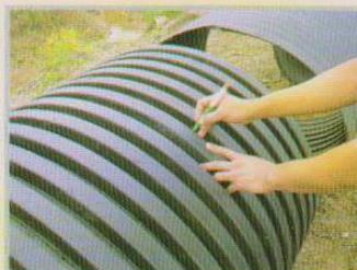
Mark the full depth of insertion on the spigot.
