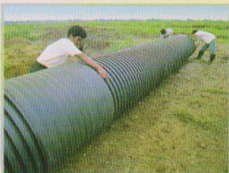
Rotate the other pipe into the coupling.
