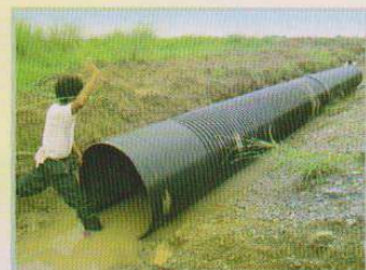
Align the pipeline properly before backfilling.
