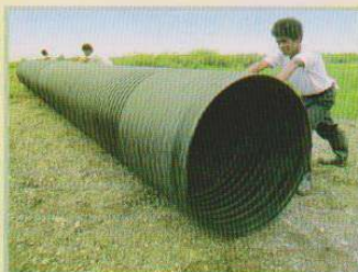
Roll the assembled pipeline into the trench.
