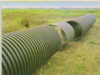
Lay the pipes along the trenchline.
